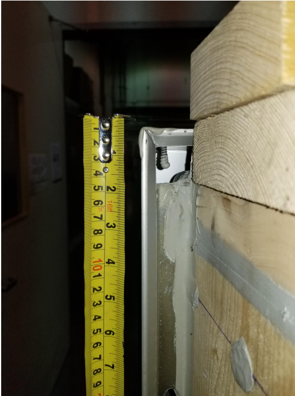
Figure 3: Exterior flashing corner fastener and sealant.
