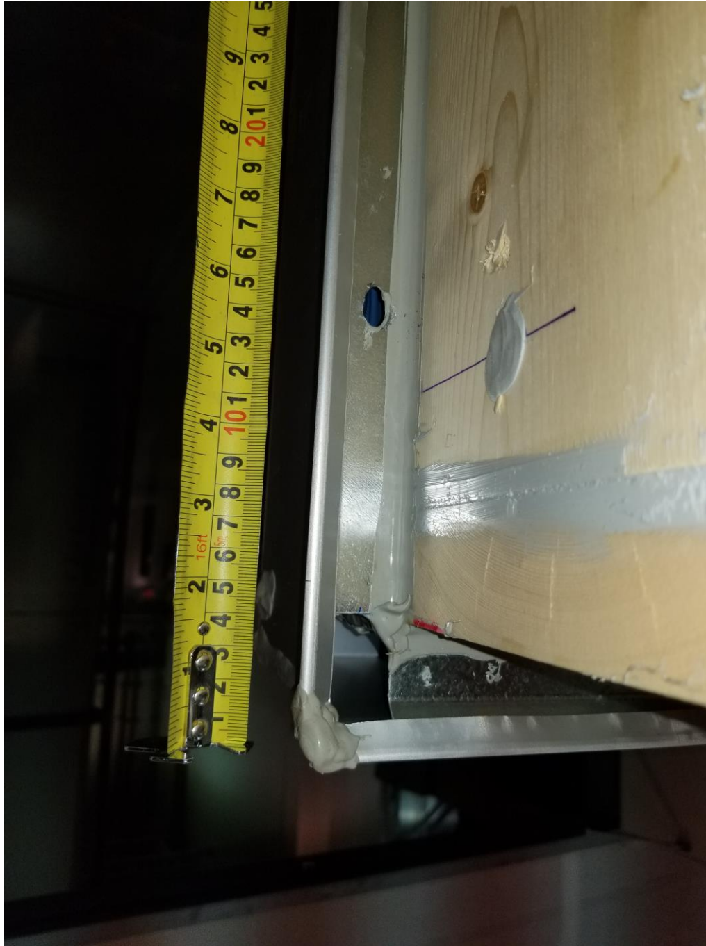
Figure 5: Exterior drainage at flashing corner.
